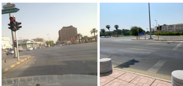
Images 17 &18: Faded road marking at crossroads
